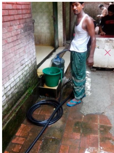
Photo 2: Water Distribution using temporary pipe from of a Public Toilet (Location: Malibagh)
